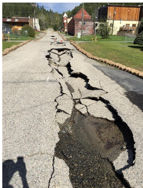
Greenwood Street Culvert Failure (May 2017)
